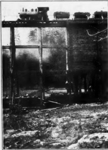
Train of Cars Over Loading Bins
